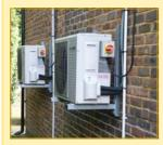
A split type domestic air to water HP is classed as precharged as the entire refrigerant charge is contained in the outdoor section. However the system still needs to be installed on site
